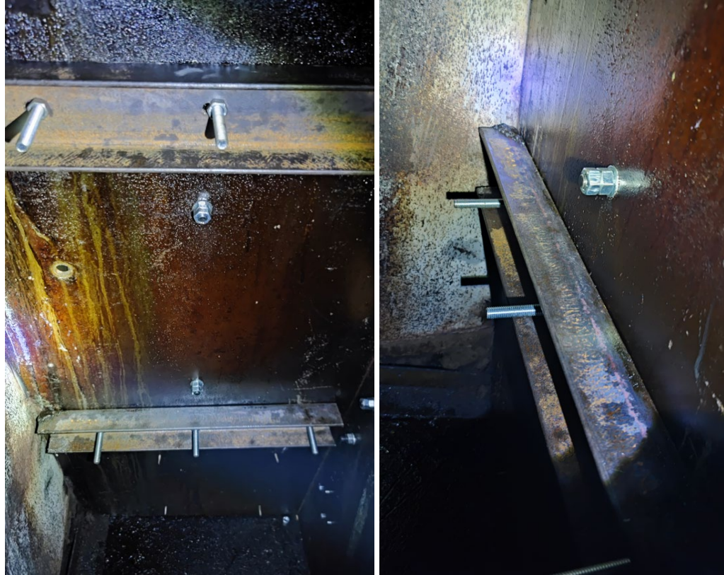
Strengthening the fan base according to the recommendations of I-care specialists.
